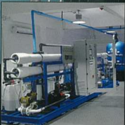
Desalination Plant for sea water
