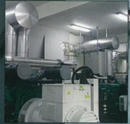
Complete Power House
