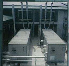
Cogeneration for hot water system
