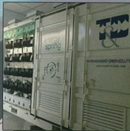
Energy Storage System
